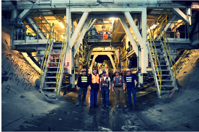
Local brothers on a tour of the Bertha Tunnel under Seattle. (Photo by Aubrey Abbott)
