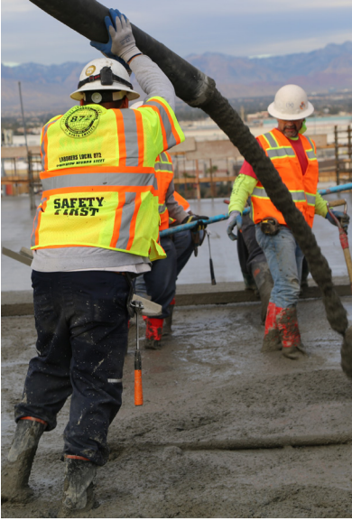
A brother from Local 872 working in concrete. (Photo courtesy of Local 872)
